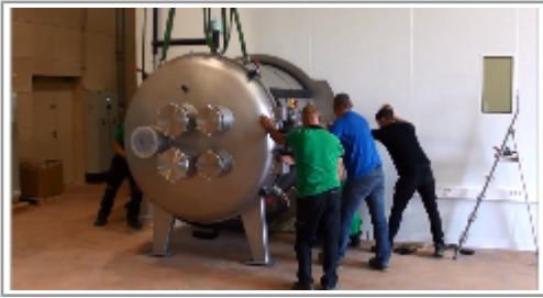
PIT VACUUM CHAMBER DELIVERY
